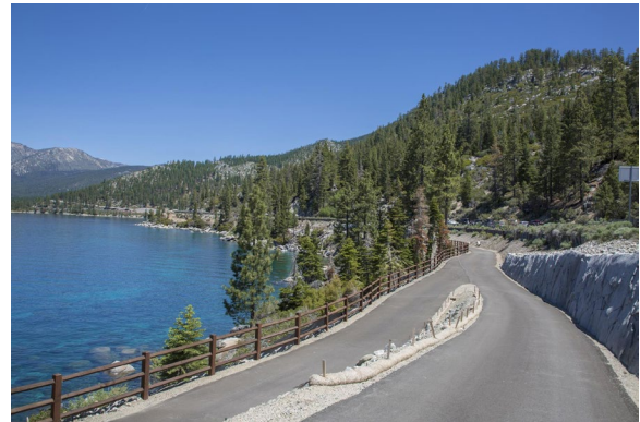
State Route 28, Incline Village, Nevada (Source: Nevada DOT)
